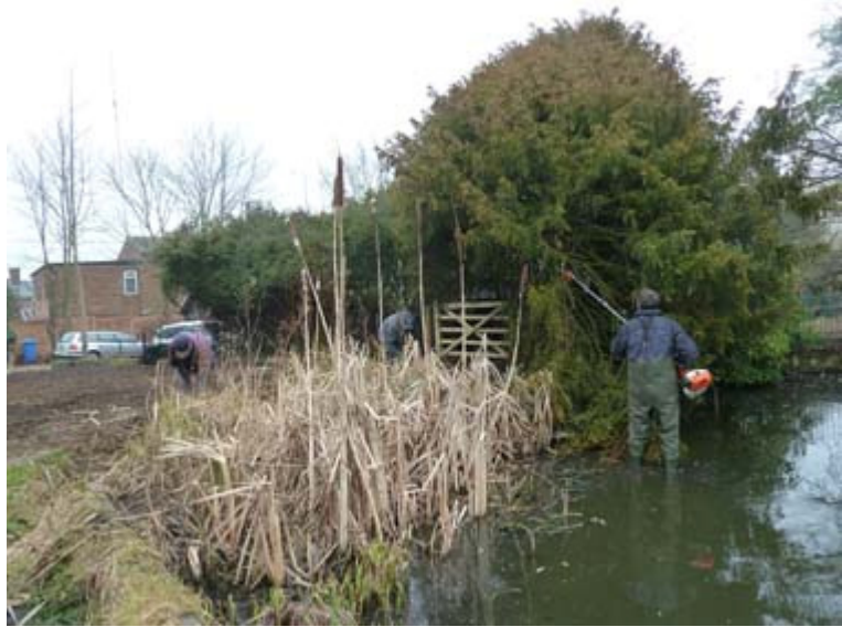
Cutting back tree growth on Foundry Pond
